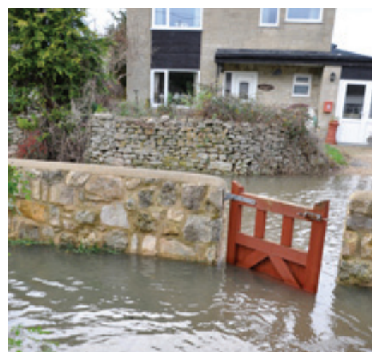
Major flooding in November 2012 saw between 500 and 800mm of flood water engulf South Hinksey
