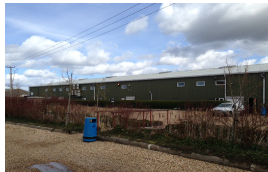
The warehouse requiring a hard wearing flooring refurbishment
