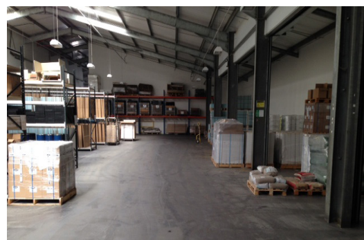
Newton 701 was easily applied and fast curing enabling a fast project turnaround.
