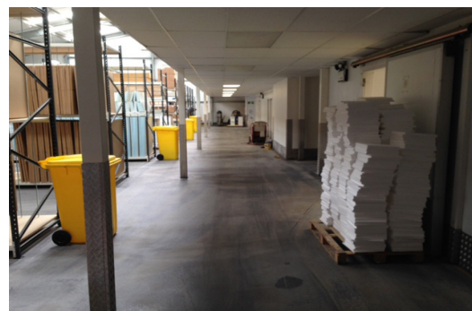
Newton 701 High Build Epoxy coating applied to the floor.
