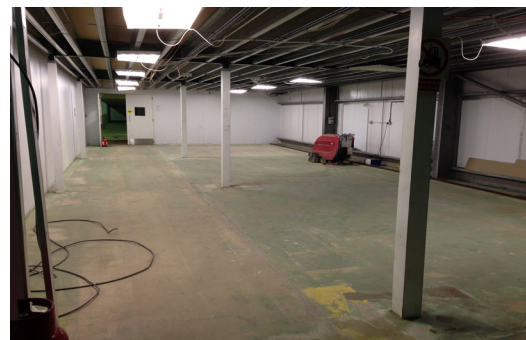
A new floor coating was required to withstand heavy forklift traffic
