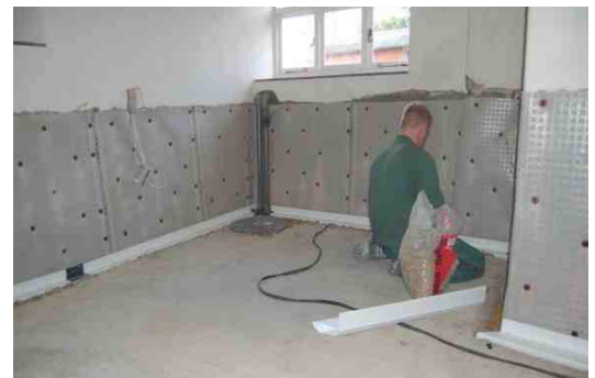
Newton 508 Mesh and Basedrain installation
