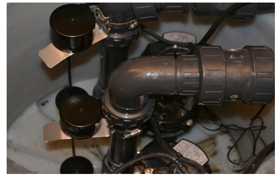
Installation of the Newton Dual Pumping System, comprising two NP750 Pumps
