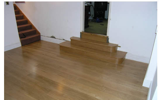
The damp proofed oak floor installed over Newton 603
