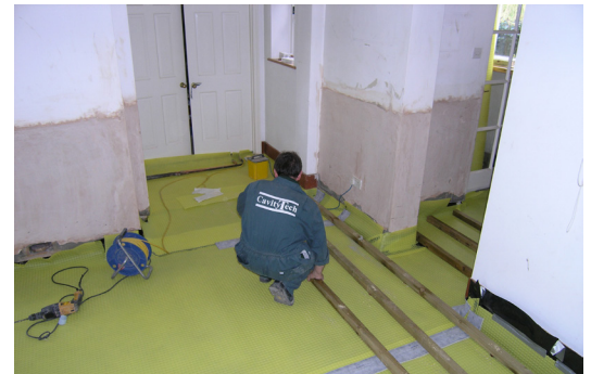
Newton 603 installed over the original damp concrete slab
