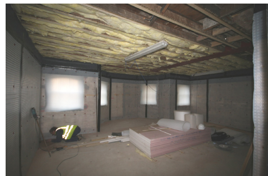
Newton System 500 installation in progress
