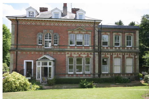
This Georgian Manor House had a 15 room basement requiring waterproofing
