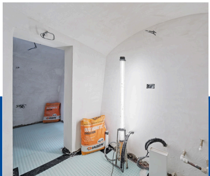
The finished internal space is now completely dry and usable
