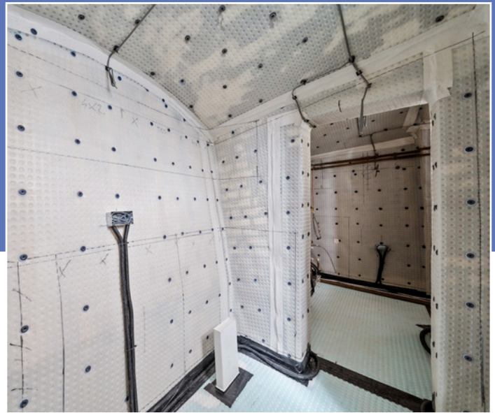
Newton 508 Mesh was installed throughout the Listed basement
