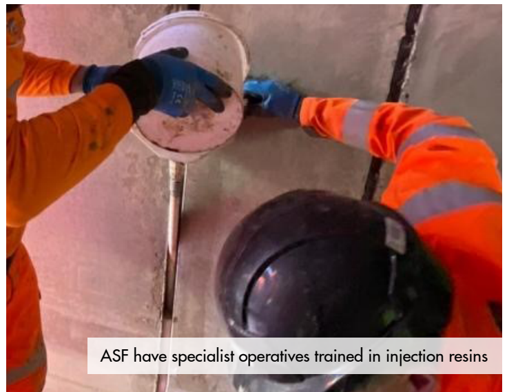
ASF's operatives prepare the resin before application
